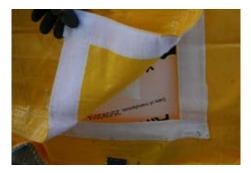
7. On full inflation of the AirDeck, make sure that the liner does not protrude and that the flap will close fully to protect the liner.
