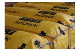
10. Cover the whole floor area. Clip the last bag in the row to its neighbour before inflating further bags. If necessary, partly inflated bags can be squeezed in to small or awkward gaps.
