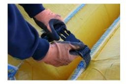
9. Add more bags by following Steps 1-7 and clip them together. If the bags are not constrained by outer walls and are being used in an open situation, use bags with clips both top and bottom to ensure no movement of the bags.
